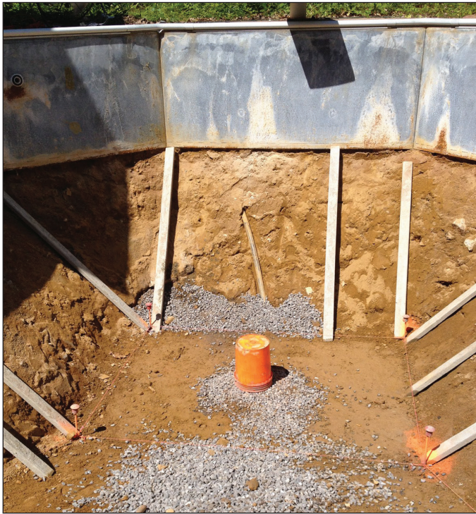
Refurbishing an in-ground pool with a new, insulating, perlite-concrete pool bottom.
